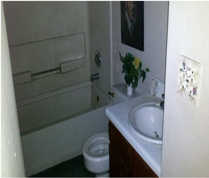
Bathroom before – Filthy tub surround, decayed subfloor, Rotted vanity, cracked sink
