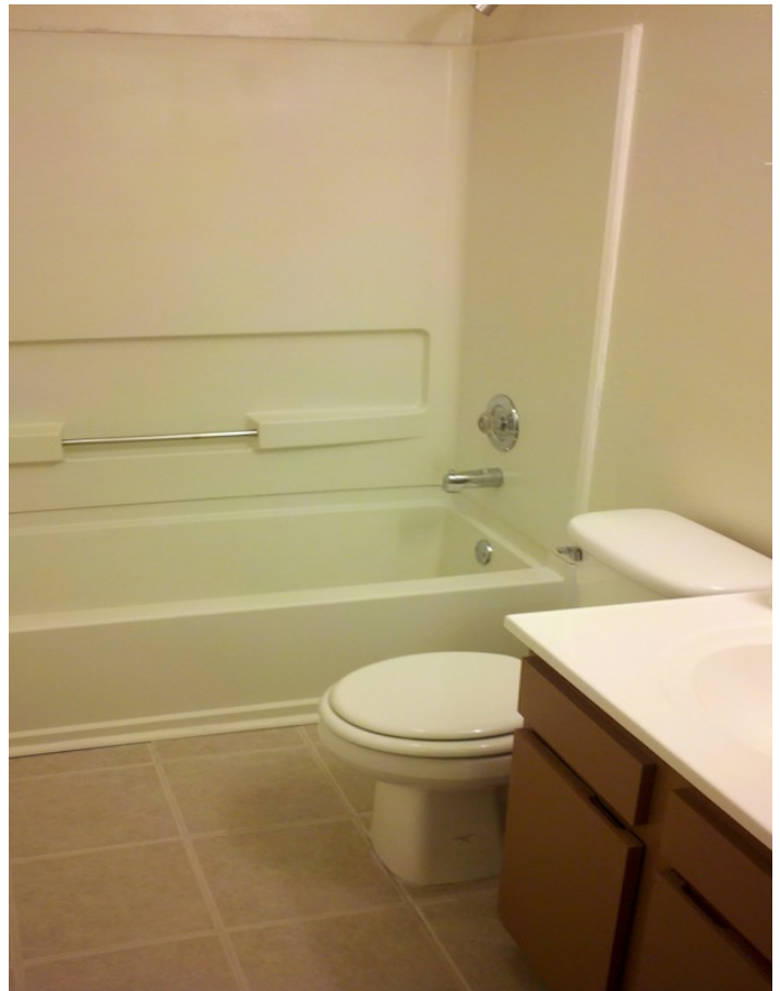
Bathroom after – cleaned tub surround, Replaced subfloor, new tile, new vanity New sink, new fixtures, new toilet
