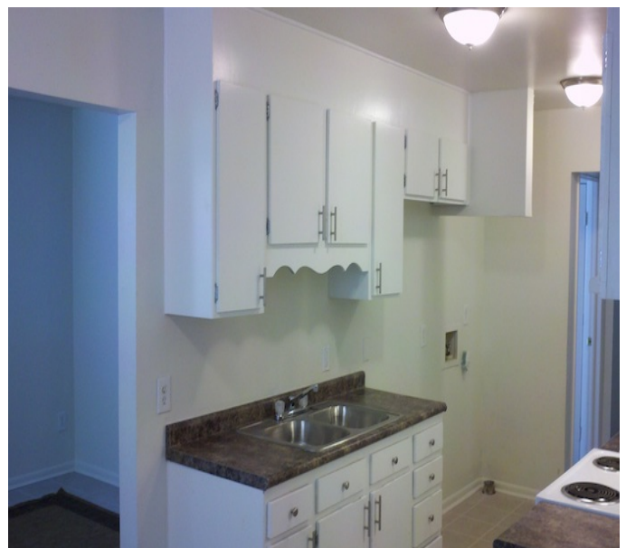
Kitchen after - repaired and painted cabinets, new hardware, new counters, new sink, new upper cabinets over stove, new washer/dryer area, new tile
